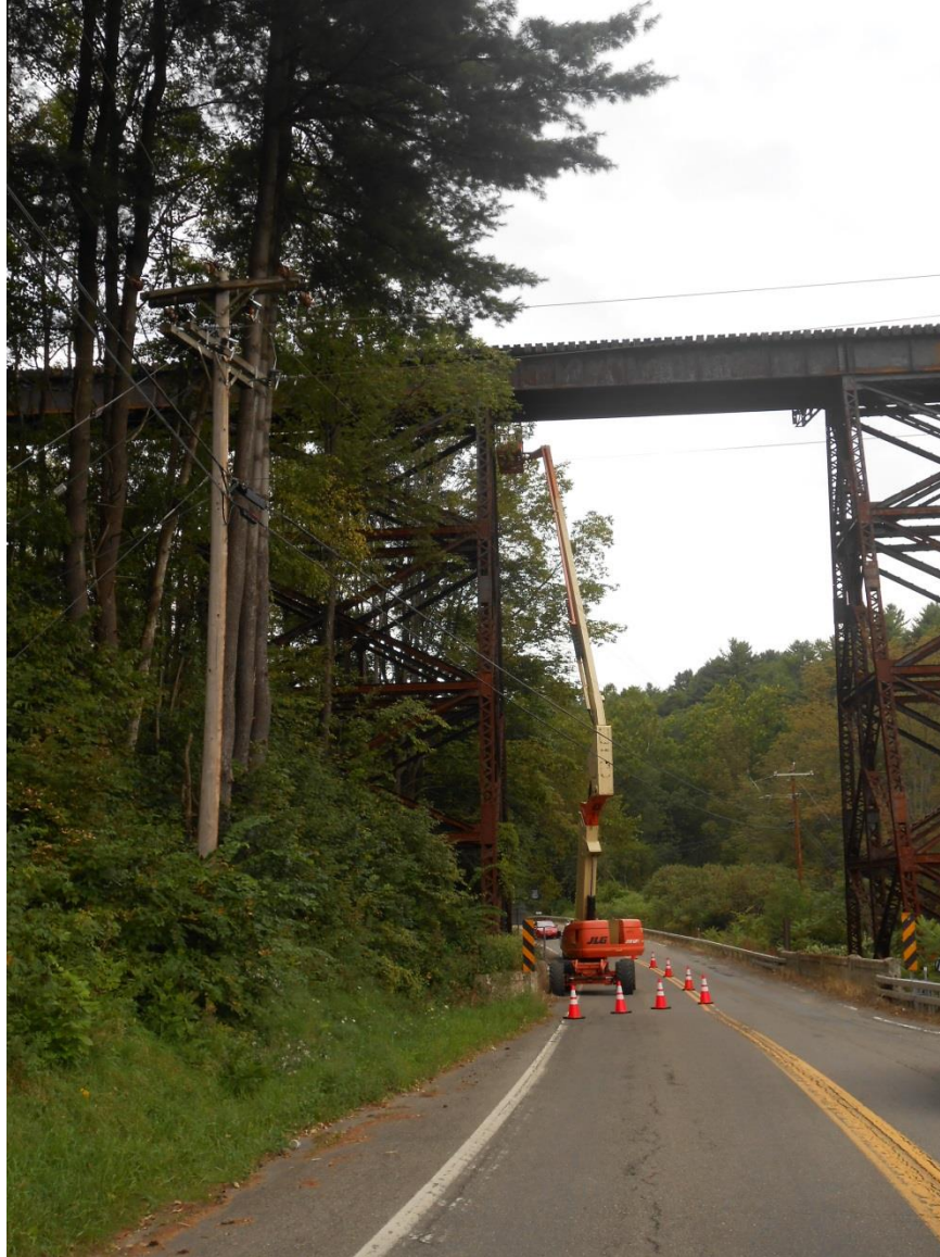
Figure 5. Telescopic boom lift and railroad bridge.
