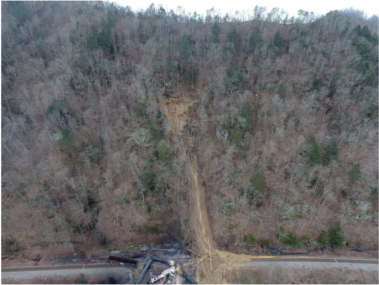
Figure 2. View of the derailed cars and the mudslide.
