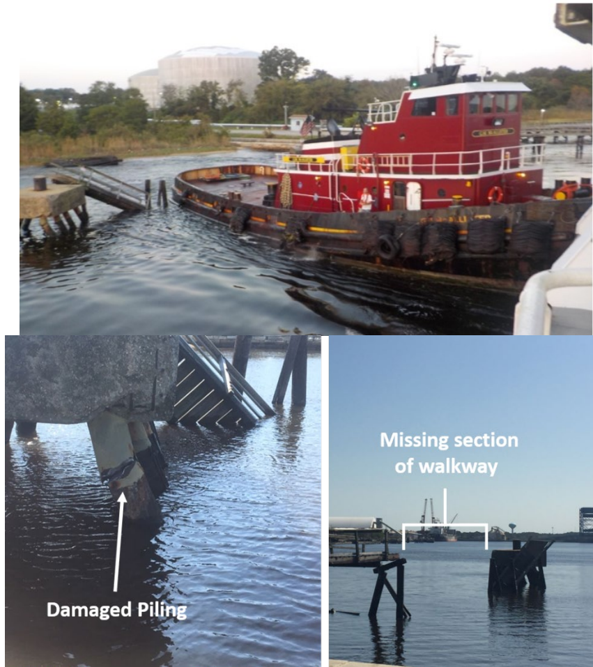
Top: G.M. McAllister at the NGL Energy Partners berth immediately after the accident (Source: Master, Ijssel Confidence ). Bottom left and bottom right: Damaged NGL Energy Partners berth after the accident (Source of right photo: US Coast Guard).
