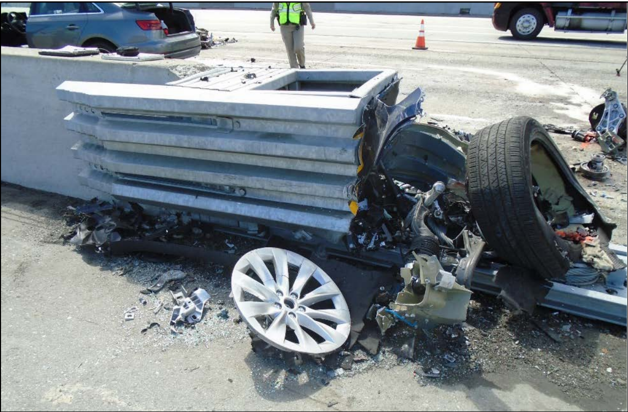
Figure 2. Postcrash photograph of the damaged crash attenuator with vehicle components lodged inside its hollow interior section. (Source: California Highway Patrol)
