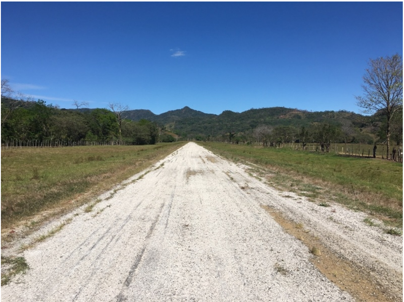
Figure 2 - View from runway looking north toward the mountains
