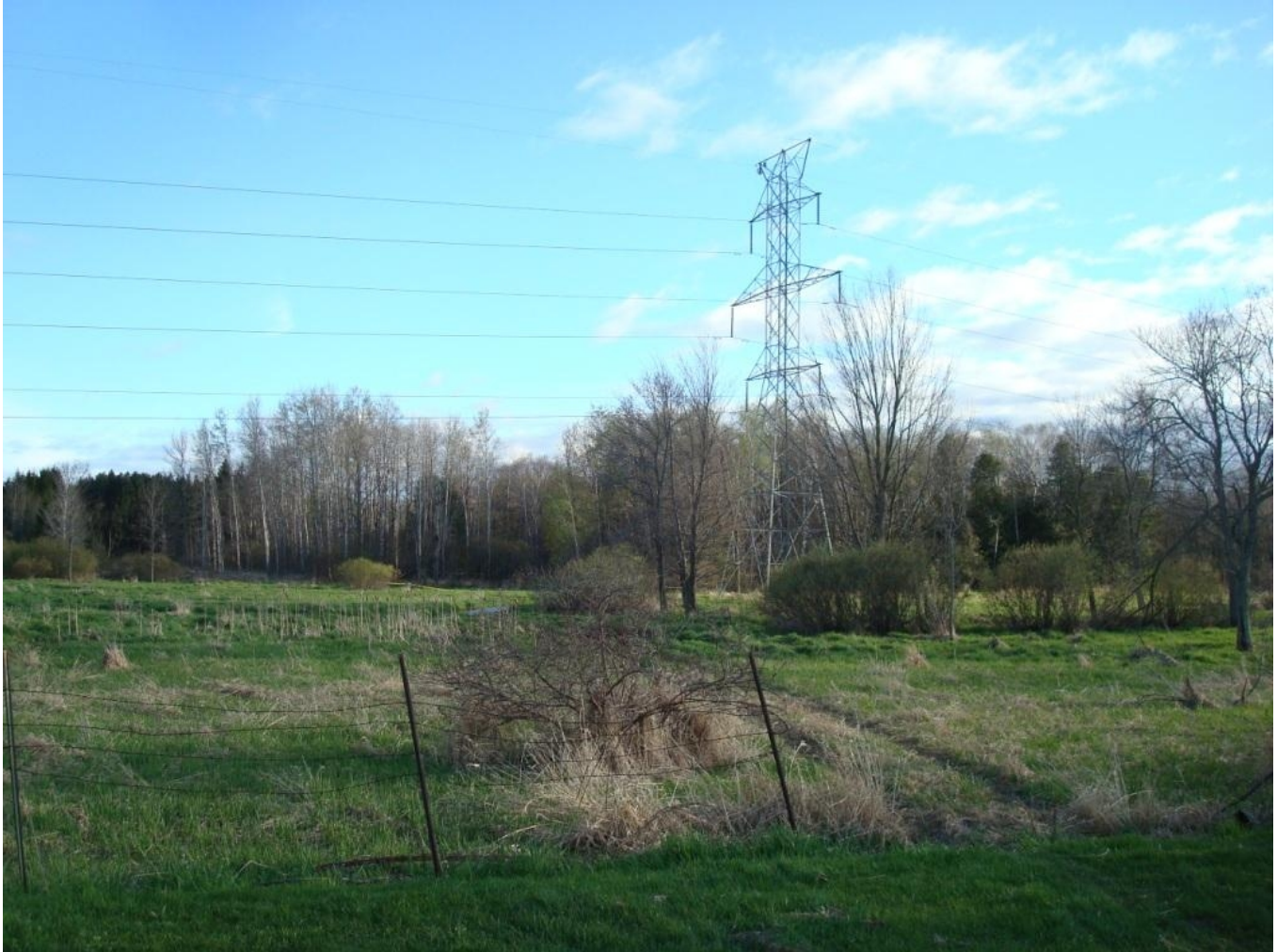
Figure 2 – View from project employee witness location, facing south toward tower 9904
