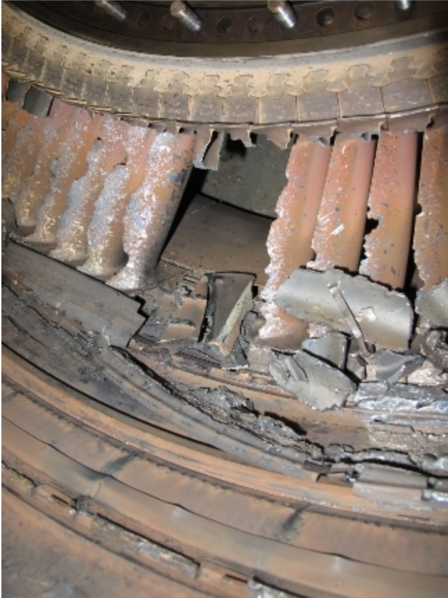
Photo No. 2: View of missing 3rd stage turbine vane cluster with piece of 3rd stage turbine vane cluster inner shroud lying in bottom of engine in location of missing cluster. (P&W)
