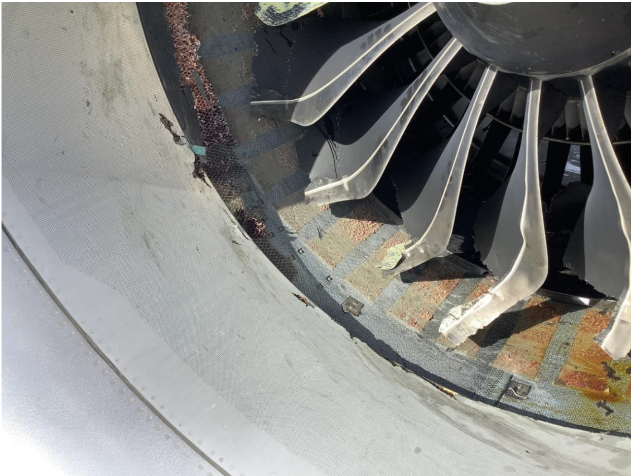
Figure 3. Close-up photo of damage to the left engine. (Source: Southwest Airlines)
