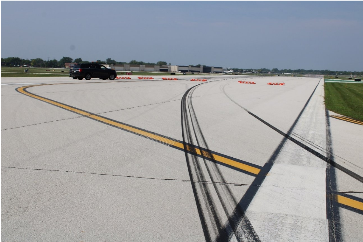
Figure 2. Airplane tire skid marks (Source: Airport operations).
