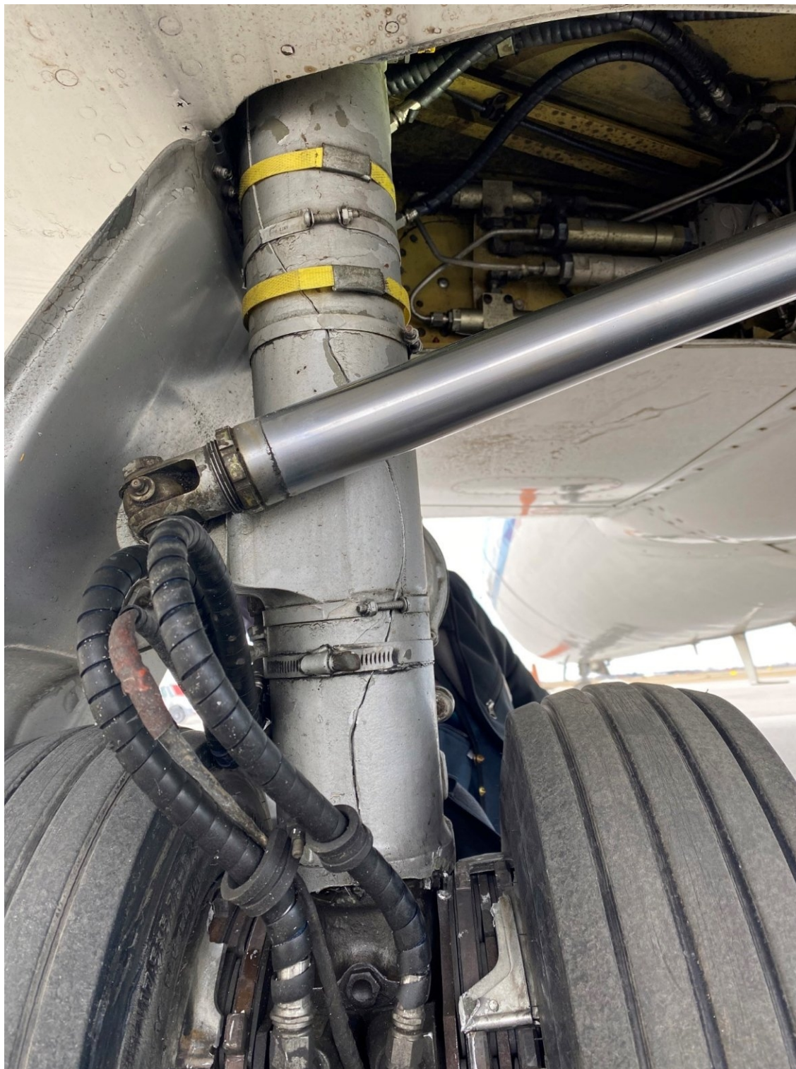
Figure 2 - View of Fractured Landing Gear Leg and Fractured Brake Caliper Retention Caps
