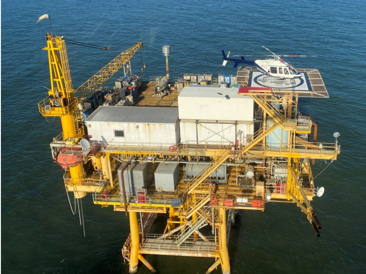
Image 1 – Overview photo of West Delta 106 platform with exemplar Bell 407 helicopter on the helipad. The helicopter is facing southeast on the helipad. The damaged chain link perimeter skirt on the southwest side of the helipad was removed after the accident.
