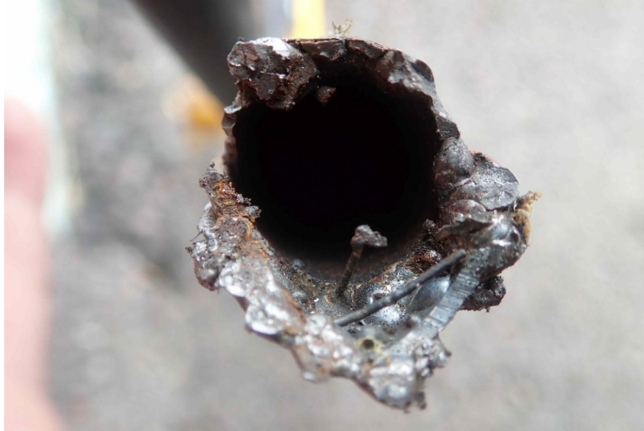
Figure 3 – Incomplete weld of left lower wing box longeron
