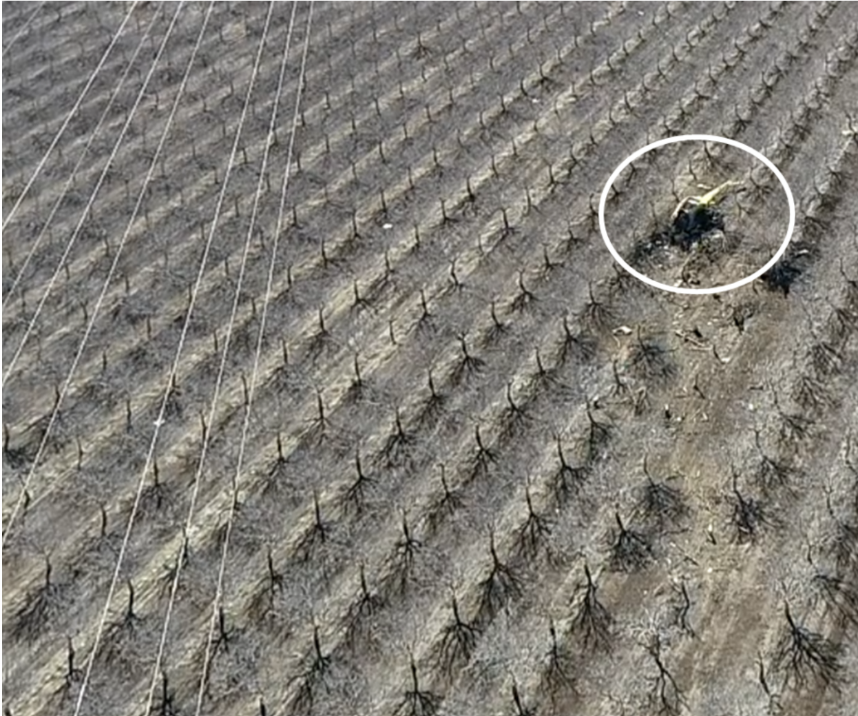
Figure 2. Aerial view of the accident site and the power distribution lines (left side).
