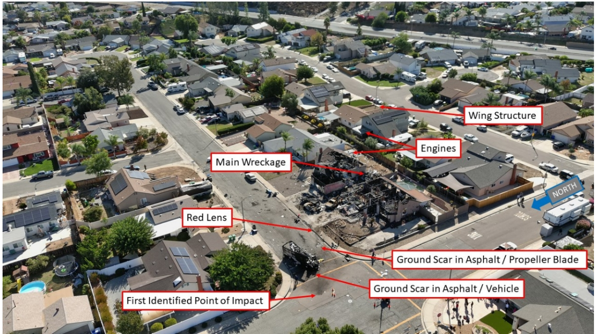
Figure 3: Annotations of wreckage locations. Aerial photo provided by San Diego County Sheriff.
