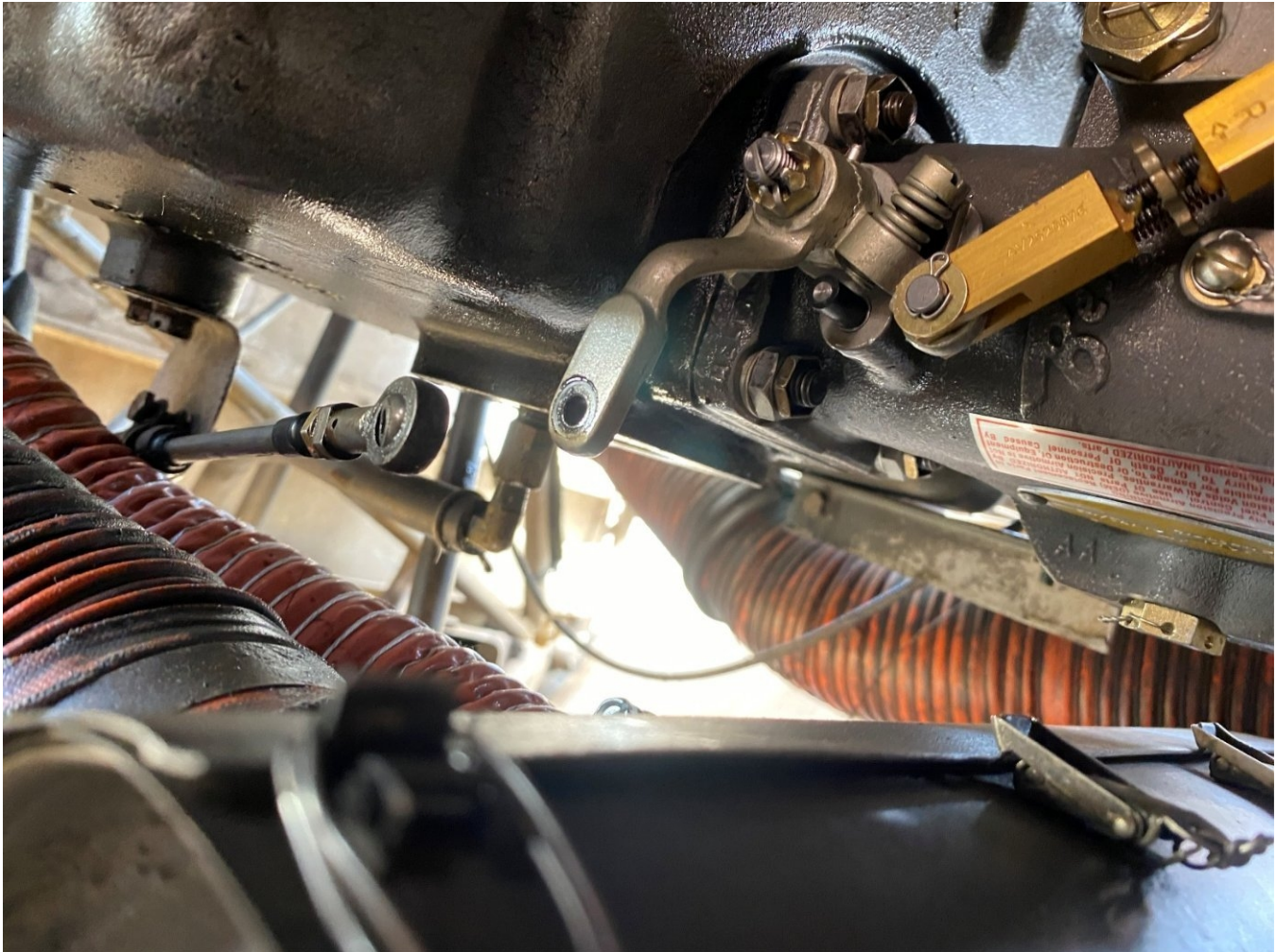
Figure 1. Throttle control rod-end found disconnected from the fuel servo throttle linkage.
