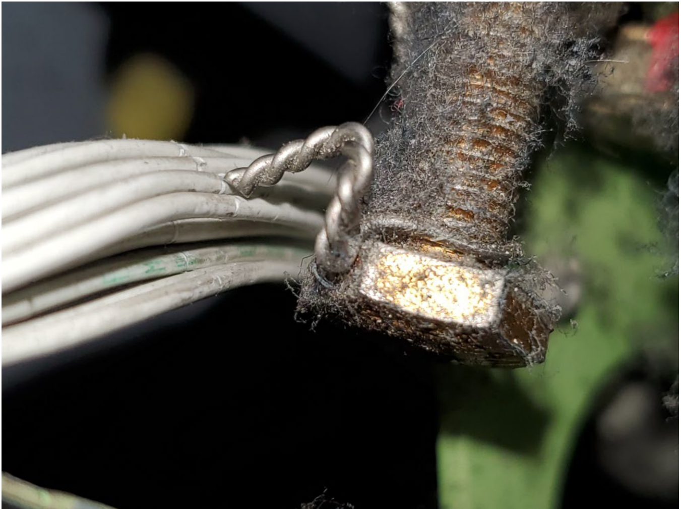
Figure 2. Bolt with pigtail contacting wires (Source: Republic Airways).
