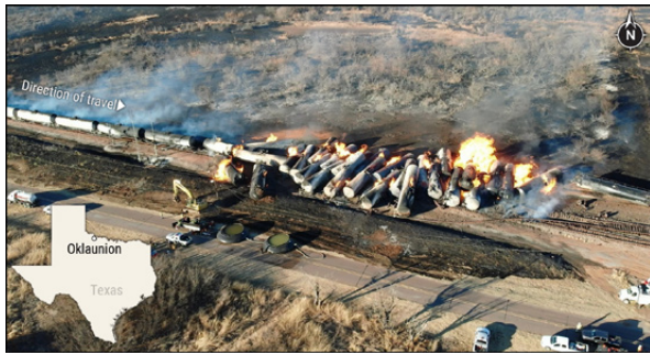
Figure 33. Aerial view of the derailed train and pool fire at the accident scene in Oklaunion, Texas. SOURCE: BNSF RAILWAY COMPANY
