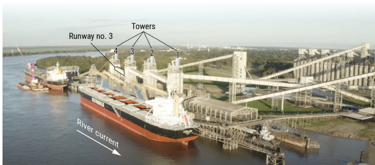
Figure 60. The ZGC shoreside facility before the accident. An unknown vessel, similar to the GH Storm Cat , is pictured. Runway no. 3 is noted between towers 3 and 4. BACKGROUND SOURCE: ZGC
