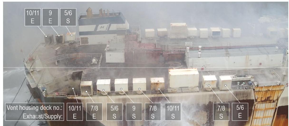
Figure 99. Damaged aft ventilation housings after the reported explosion of portside vent housing for deck 9 (9E in the photo). BACKGROUND SOURCE: JACKSONVILLE FIRE AND RESCUE DEPARTMENT
