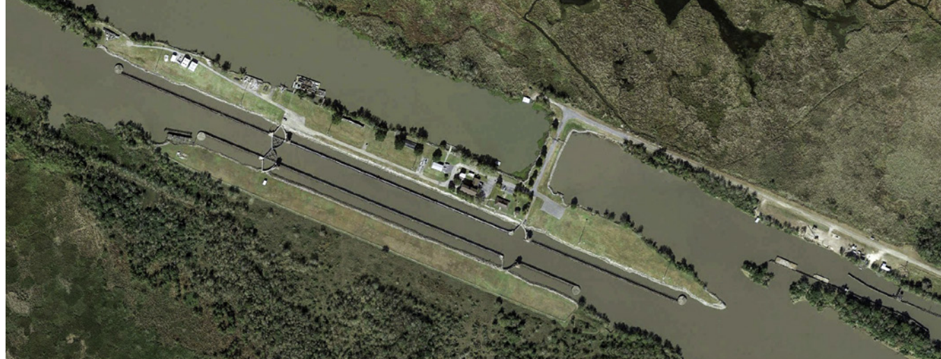
Figure 34. The Leland Bowman Lock. SOURCE: GOOGLE EARTH
