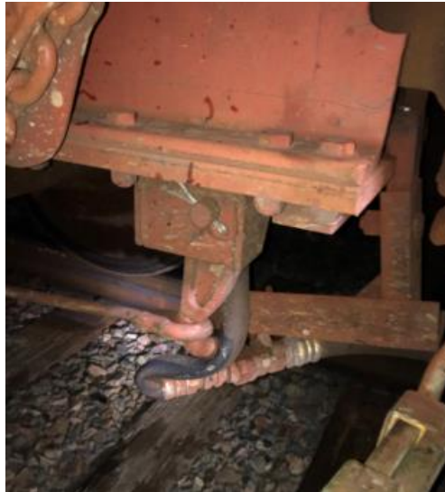
Figure 4 - Example of a kinked air hose found on a similar style freight car that was found between Cheyenne and Laramie, Wyoming after the instant accident at Granite Canyon, Wyoming ( Photo courtesy of UP )
