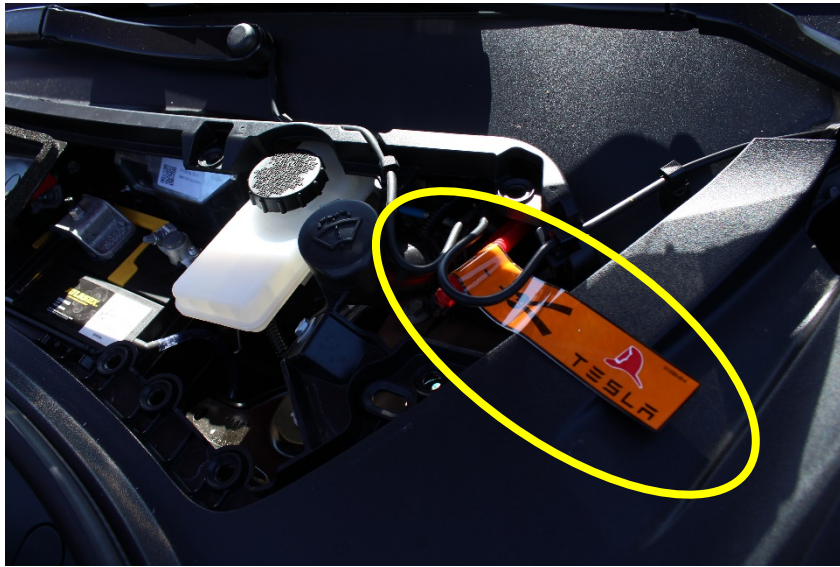
Figure 3: Photograph of the fire department tag on the power cable inside of the car's engine compartment.
