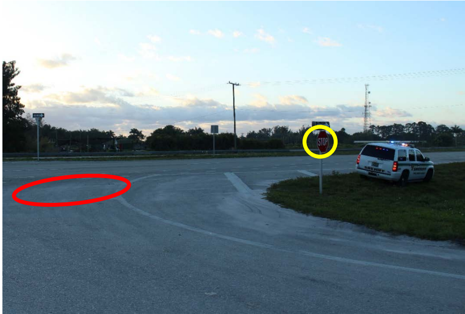
Figure 6 Photograph showing close-up of private driveway exit, stop sign (circled in yellow) and faded stop bar (circled in red). (PBSO)
