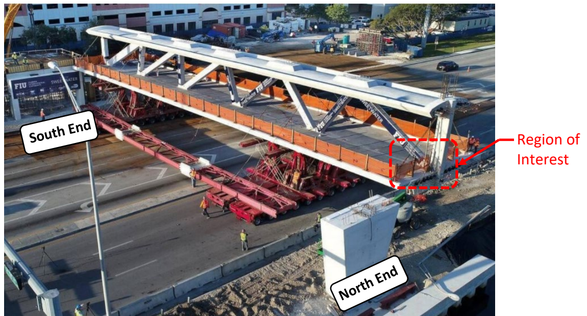
Figure 1. Main span of the bridge highlighting the portion of the bridge this is of interest to this factual report.
