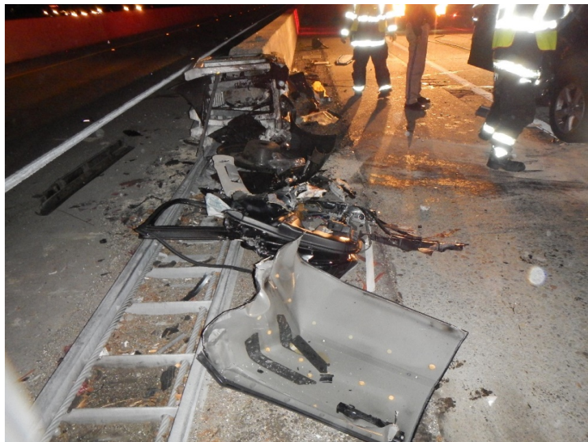
Figure 3 – Postcrash photo of crash cushion on November 14, 2015, at the exit ramp transition to SR-85.
