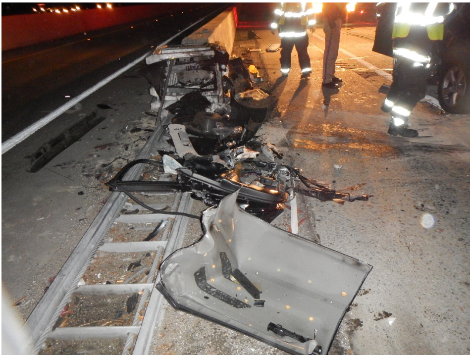
Figure 7B – Postcrash picture of crash cushion on November 14, 2015, at the exit ramp transition to SR-85.
