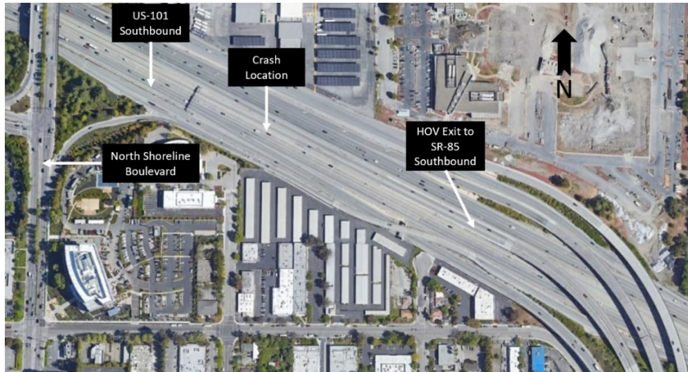
Figure 1A – Image of US-101 interchange at SR-85. (Source: Google Earth, image date March 28, 2018)
