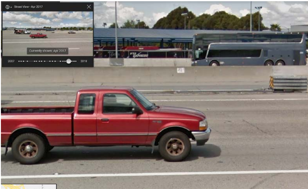
Figure 7L – Google Maps Street View image captured in April 2017 showing the crash cushion fully collapsed. Caltrans maintenance records show the crash cushion was replaced on April 14, 2017.
