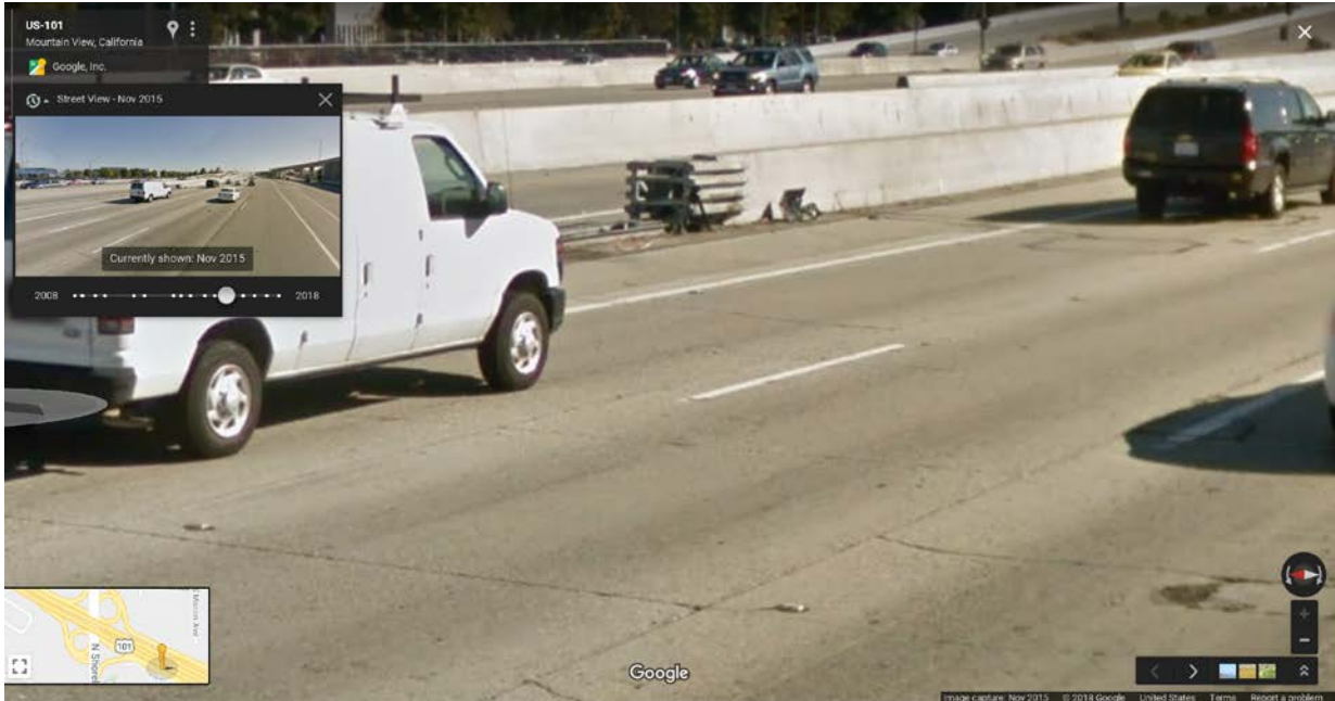
Figure 7E – Google Maps Street View image captured in November 2015 showing the crash cushion fully collapsed and missing the retroreflective object marker.
