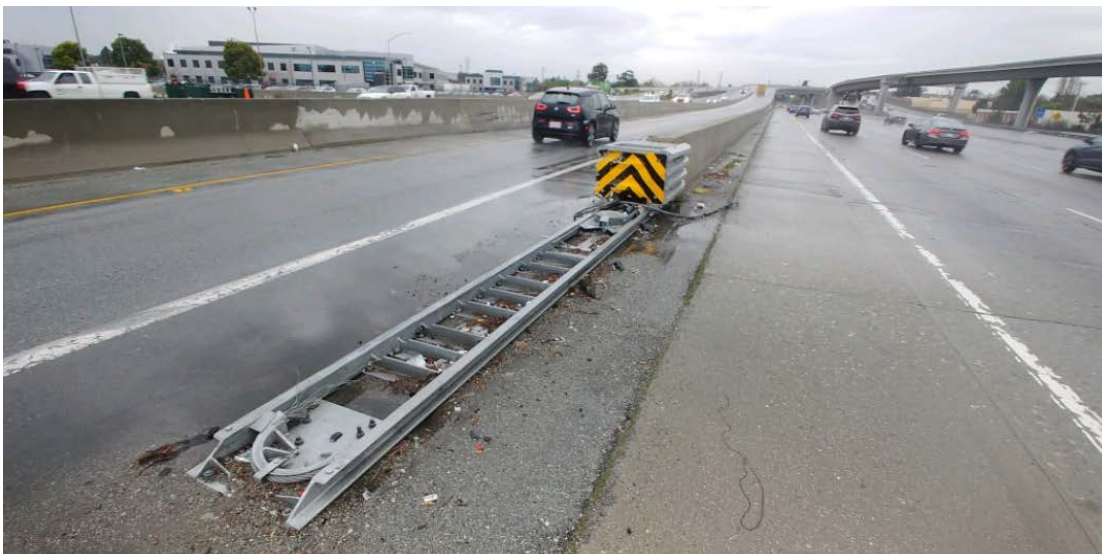
Figure 7F – Damaged crash attenuator photo taken by Caltrans worker on March 20, 2018.
