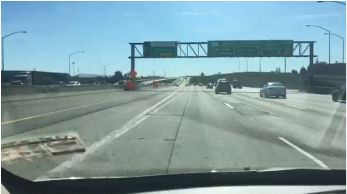
Figure 3F – Still image from video drive through at 630 feet from crash cushion. The 8-inch wide solid white channelizing line marking the left side of the gore area was the most prominent and visible.
