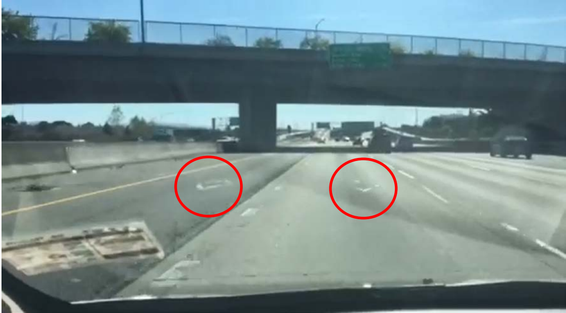
Figure 3C – Still image from video drive through at 1,365 feet from crash cushion. The painted HOV diamond symbols (circled in red) designating the two left lanes were faded and partially obliterated.
