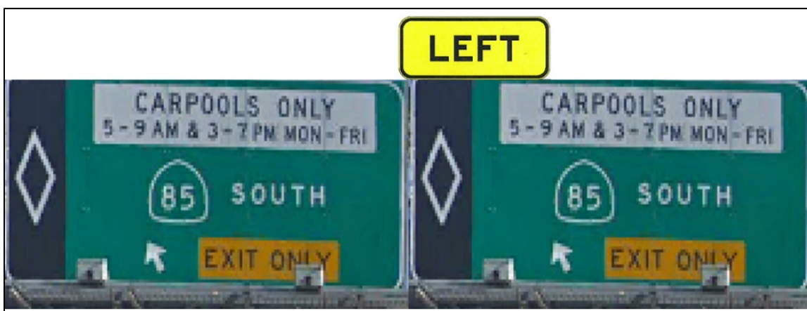
Figure 2E – Sign for left exit HOV lane at crash location (left) and example of compliant sign with required “LEFT” plaque (right).
