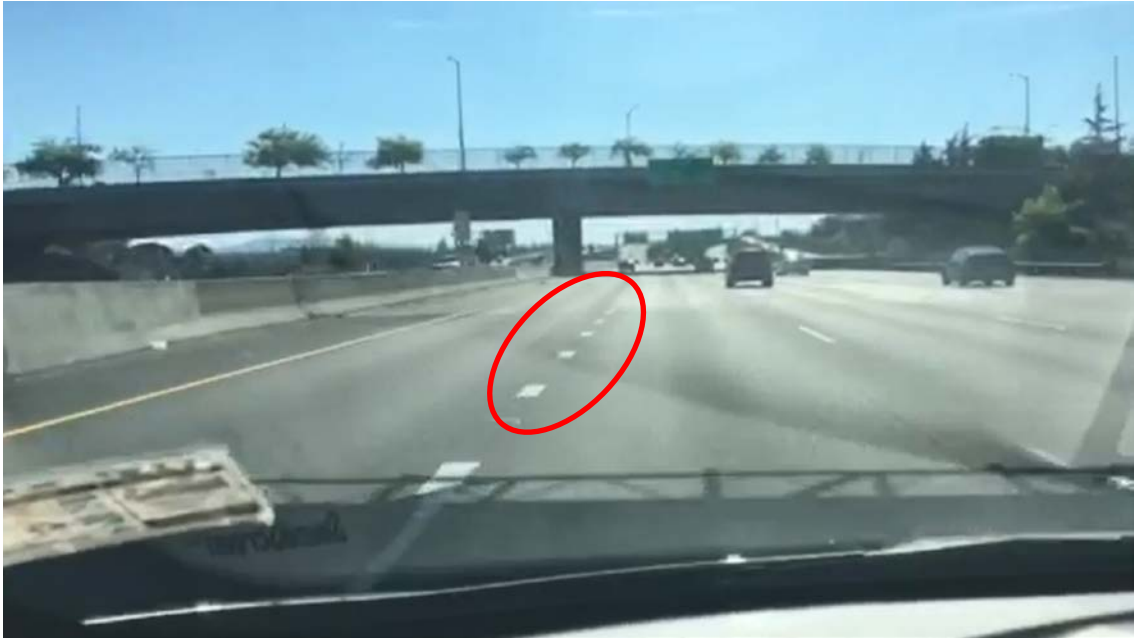
Figure 3B – Still image from video drive through at 1,540 feet from crash cushion. 8-inch wide lane drop markings (circled in red) separating the two left HOV lanes begin at this location.
