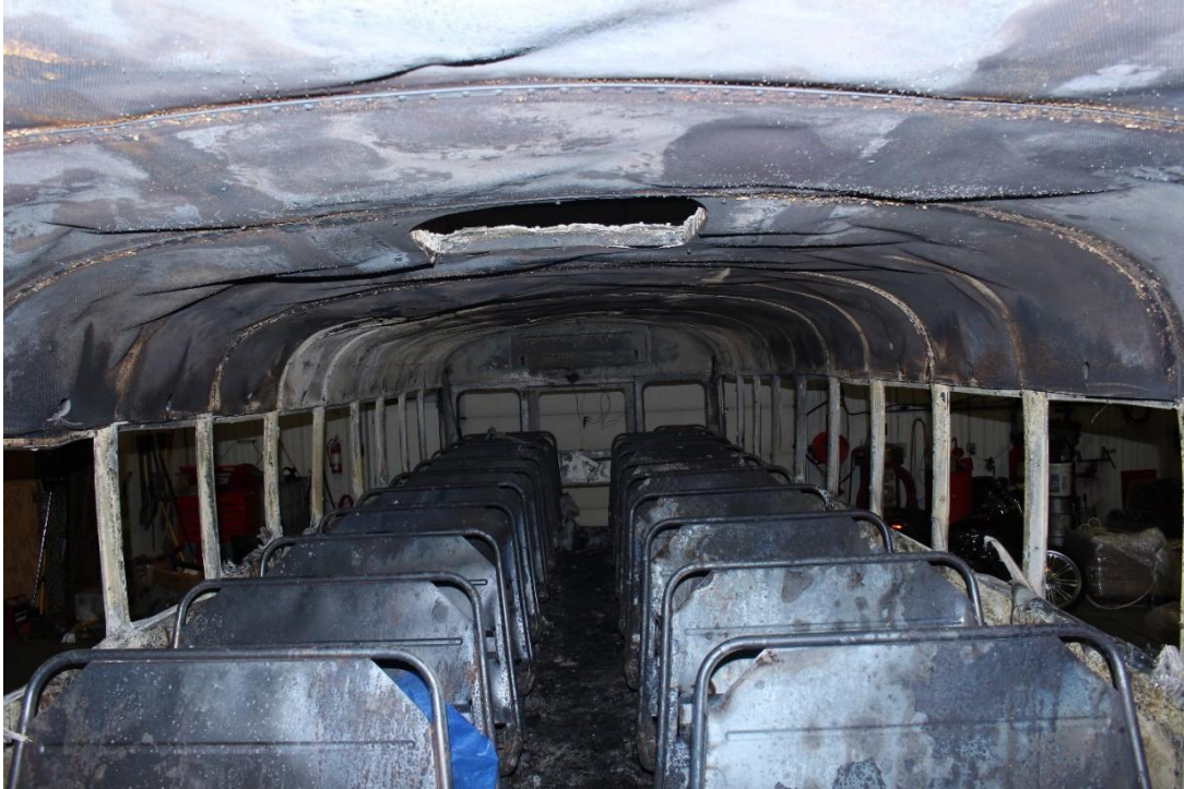
Photo #3: Interior view of damage to school bus caused by intense heat and fire.
