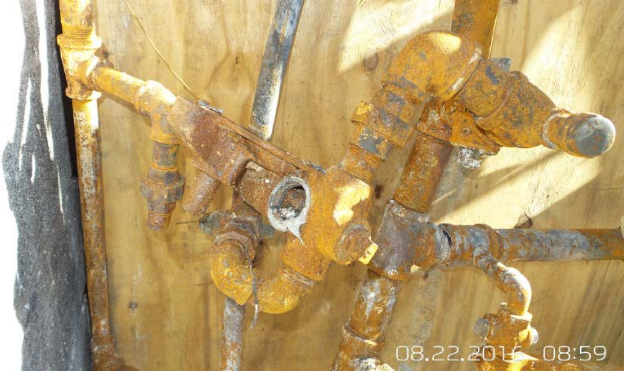
Appendix B: Photo coverage of the basement perimeter and accident area at 8701 Arliss Street by Kay Management representative.
