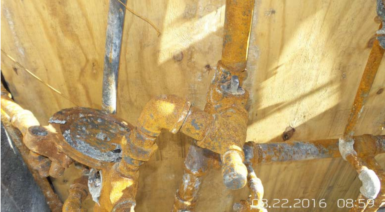
Appendix B: Photo coverage of the basement perimeter and accident area at 8701 Arliss Street by Kay Management representative.
