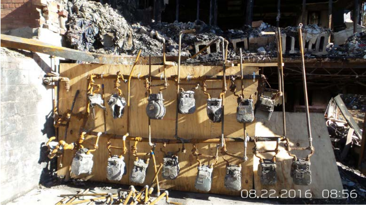
Appendix B: Photo coverage of the basement perimeter and accident area at 8701 Arliss Street by Kay Management representative.
