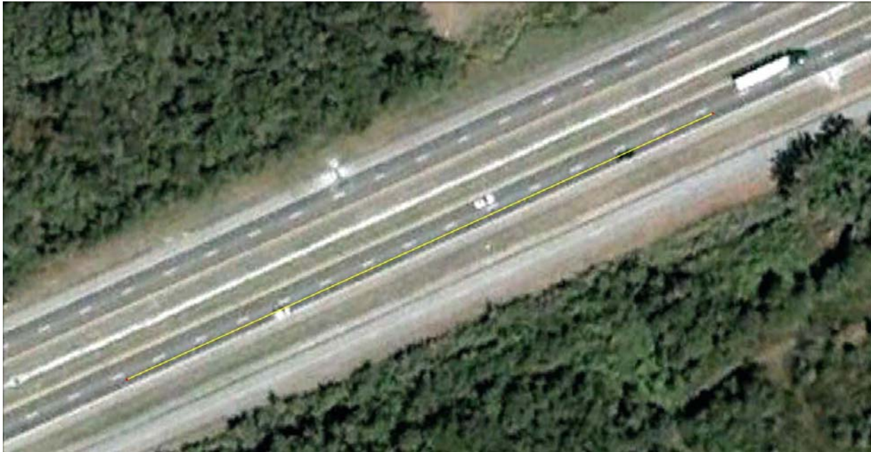
Figure 1 Google Earth Image of the Analyzed Road Segment with a Superimposed 550 ft Ruler
