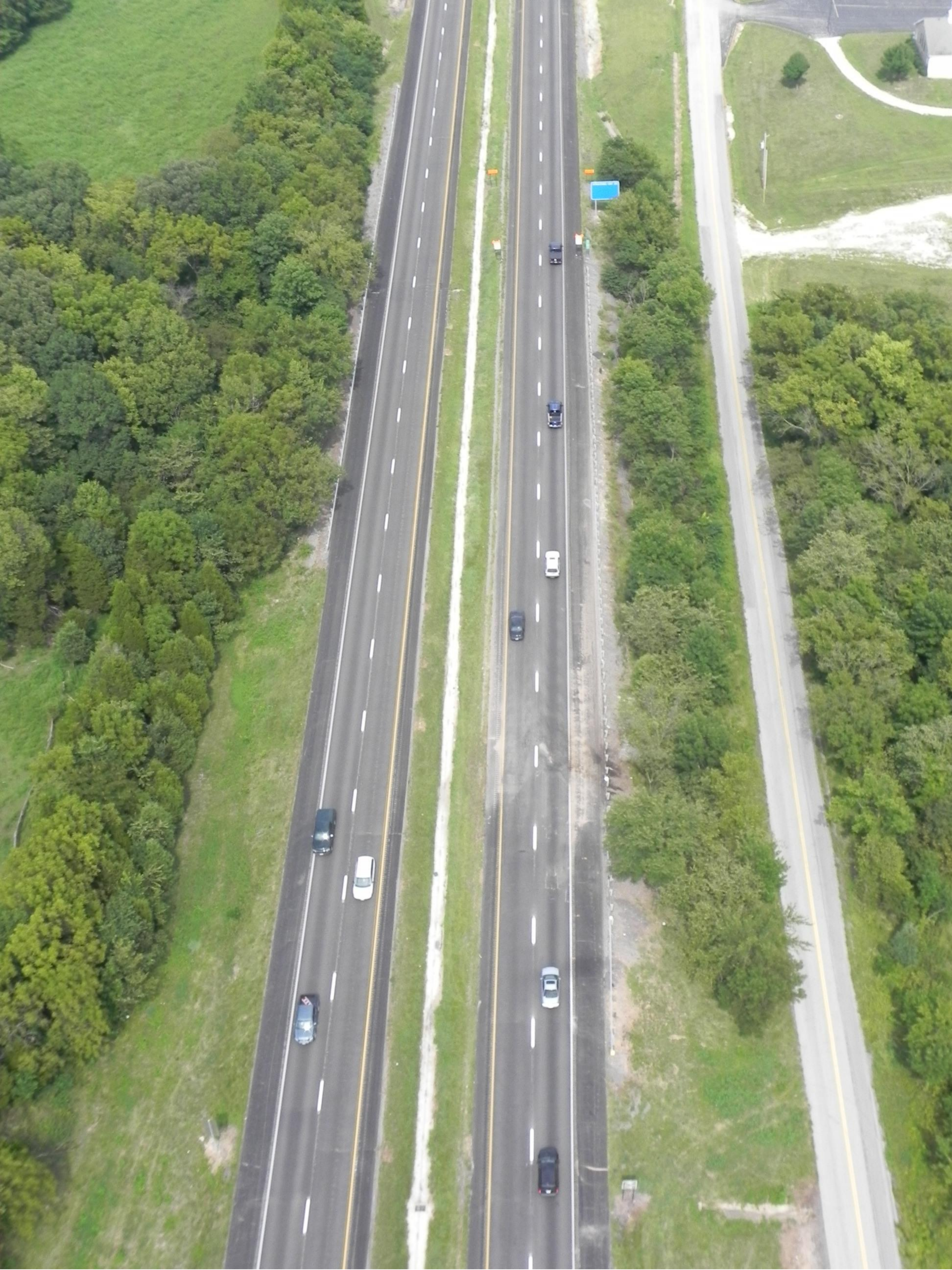
HWY Photo 31, Aerial View of Accident Location
