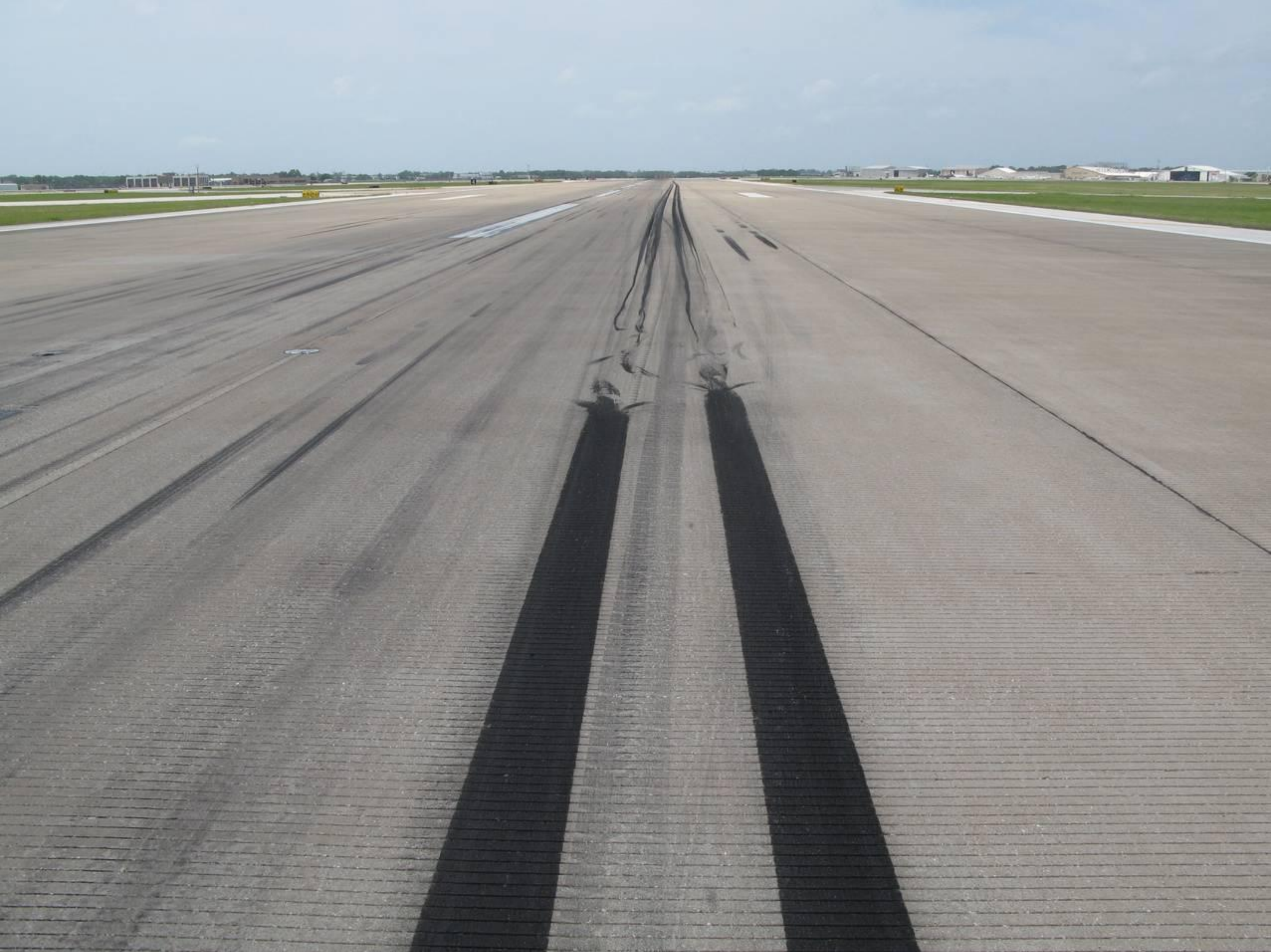
Photo 2 - Showing Marks on Runway from Both Right Main Landing Gear Tires
