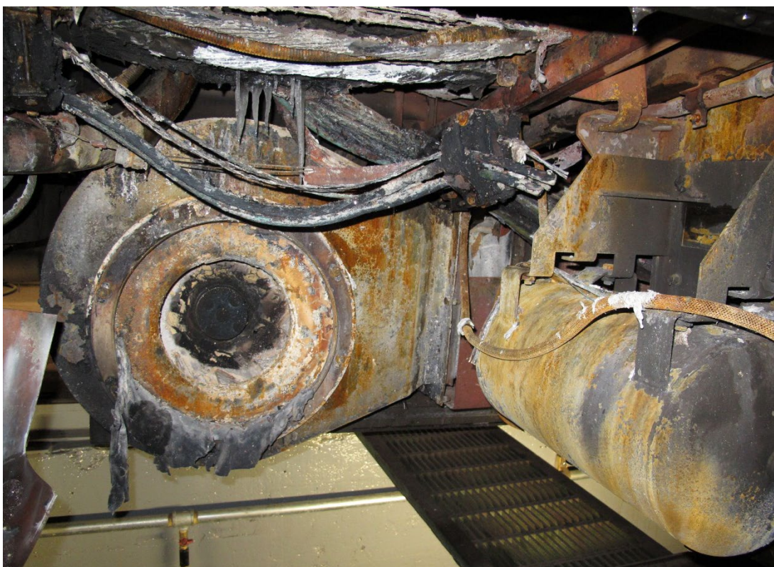
Figure 6. Undercarriage around the blowers. (NTSB)
