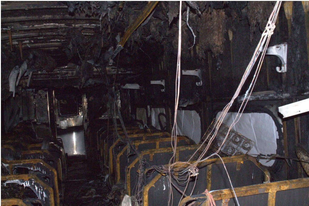
Photo 4 Interior of Car 132 showing the extensive damage caused by direct flame impingement and heat during the fire. (Source: NTSB)
