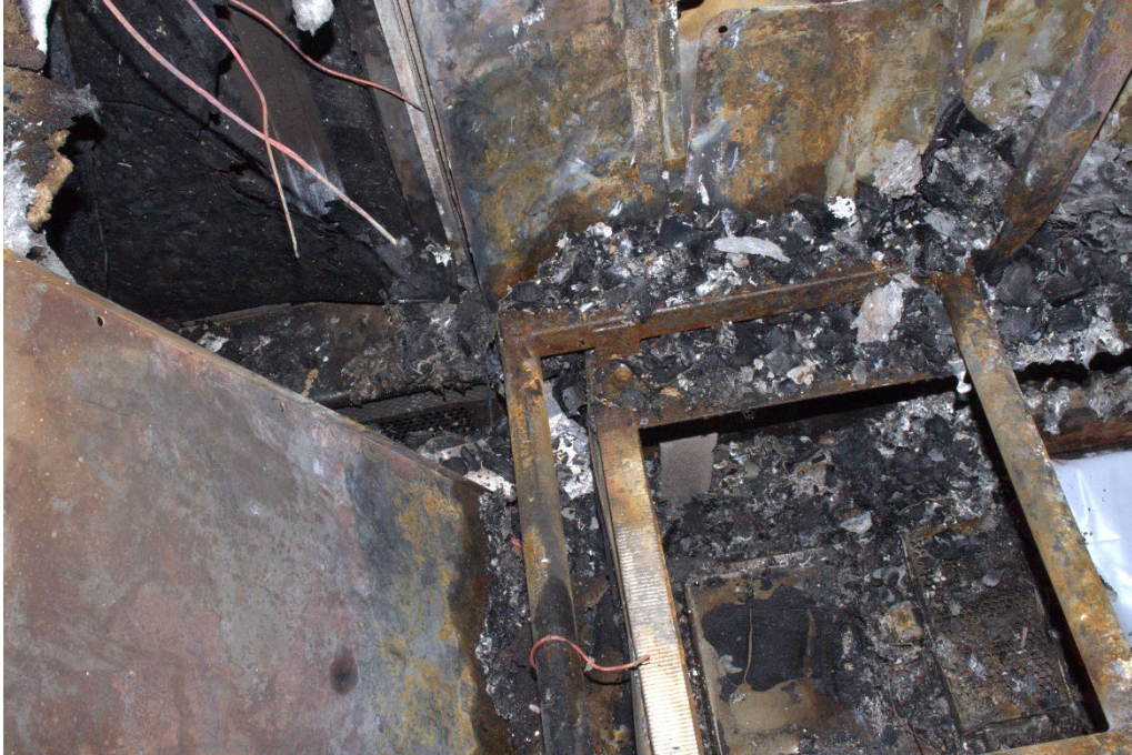
Photo 13 A closeup of the area beneath the mid-car seat where the modules were originally located after both modules were removed. (Source: NTSB)
