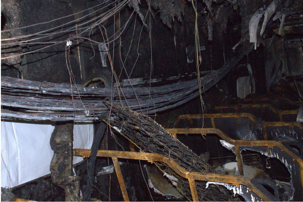
Photo 3 Interior of Car 132 and the extensive damage to the ceiling and seats caused by the fire. (Source: NTSB)
