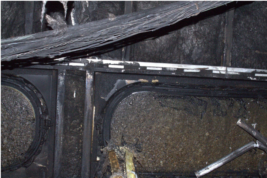
Photo 6 Closeup of the damage to the car windows still in their frames caused by the intense heat of the fire. (Source: NTSB)
