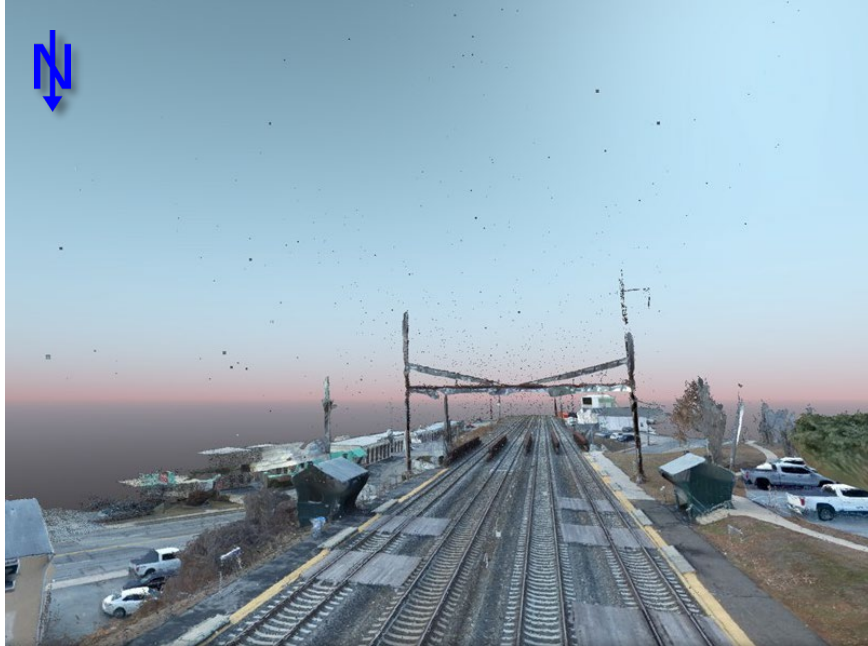
Figure 4 Screen capture of the three-dimensional point cloud of the scene shown in the direction of travel of the incident train, with the southbound Crum Lynne SEPTA train station on the right side in the foreground and the final rest position for the train in the background.
