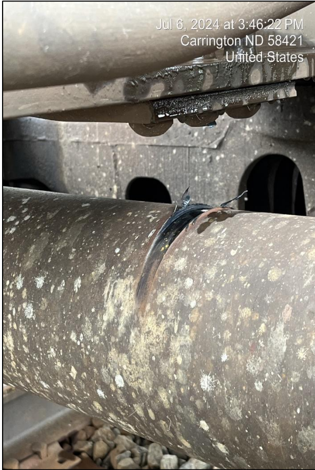
Figure 1- Exemplar photograph of the axle contacting the draft sill on car TILX500825
