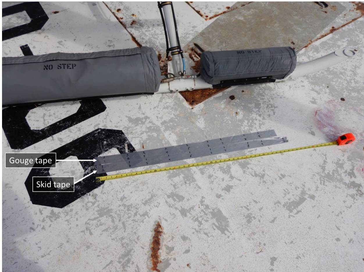
Figure 22. Photo showing the spacing of the wear shoe bolts and the paint gouges.
