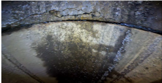
E1 Joint Location – East Pipe
