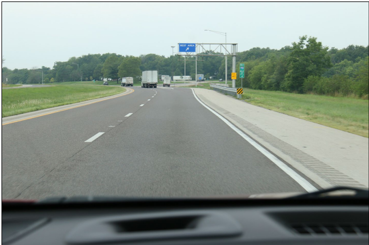
Figure 2: Photograph depicting the westbound approach to the rest area exit ramp.
