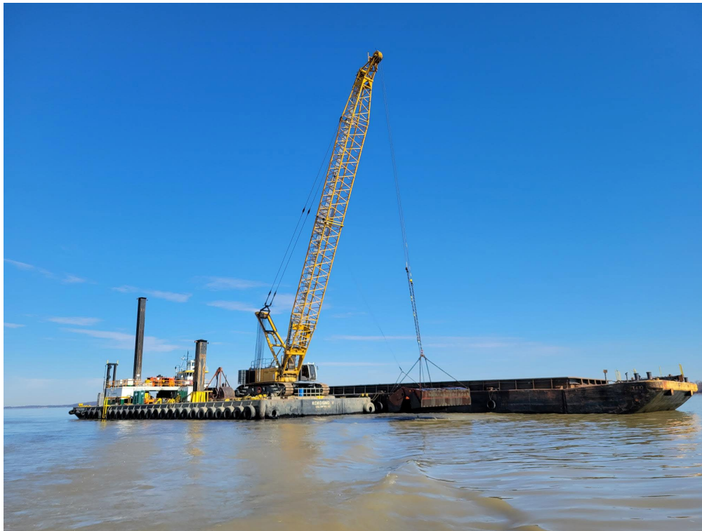
Figure 1. The barge Kokosing V , with crane. (Source: Kokosing Industrial)
