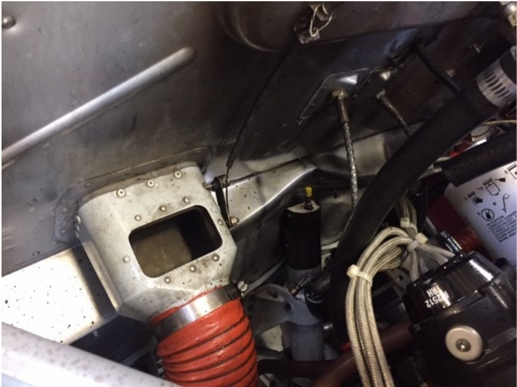
Photo 2 – Firewall Damage (FAA Photo)
