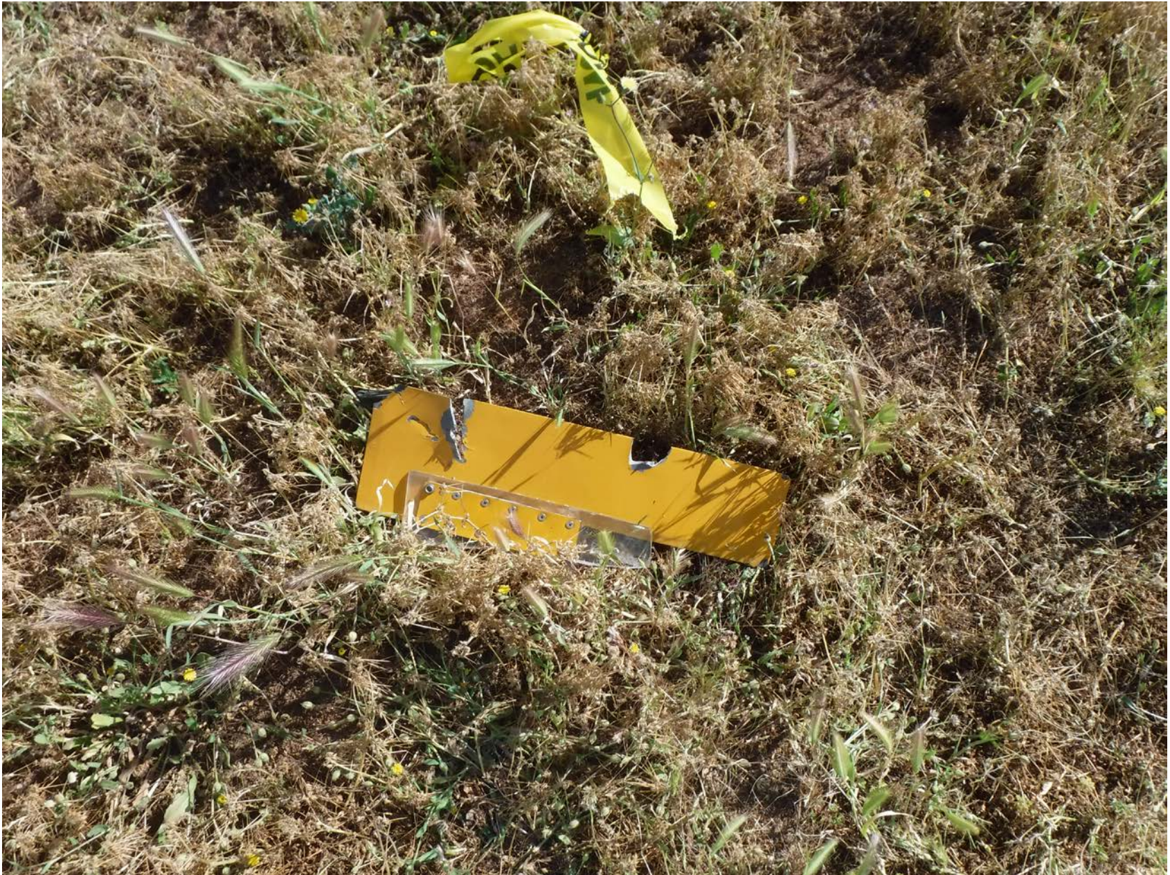
Photo 18 – Portion of canopy structure. Courtesy of California Rehabilitation Center
