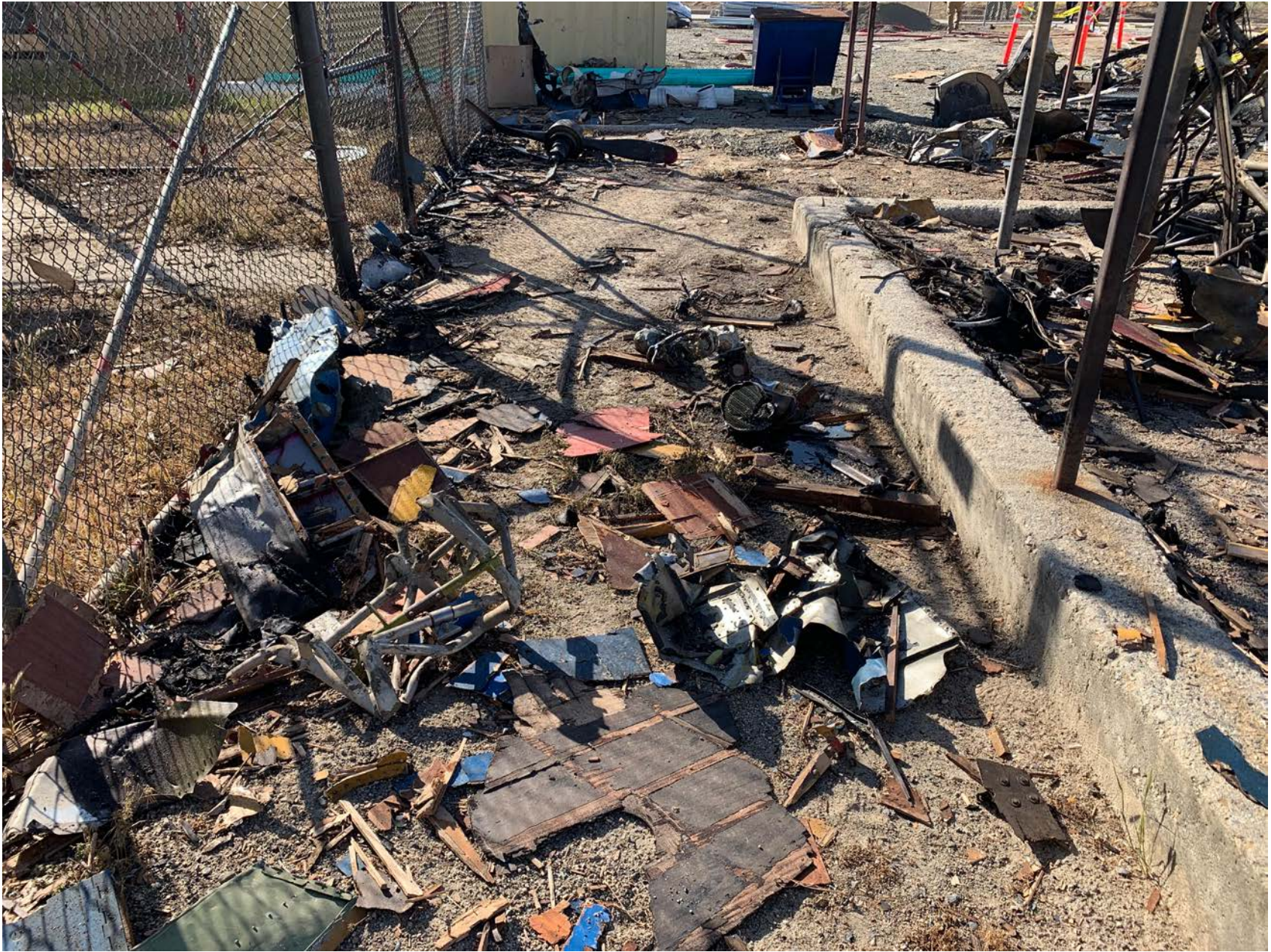
Photo 3 - View of the accident site.
