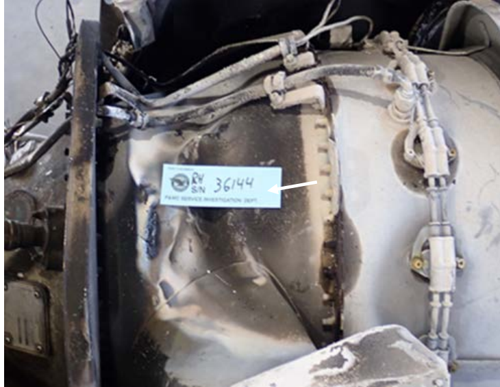
Figure 45. Exhaust duct compression damage
