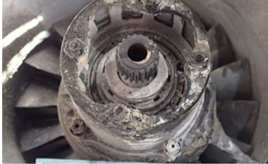
Figure 18. S1 compressor and front support bearing
