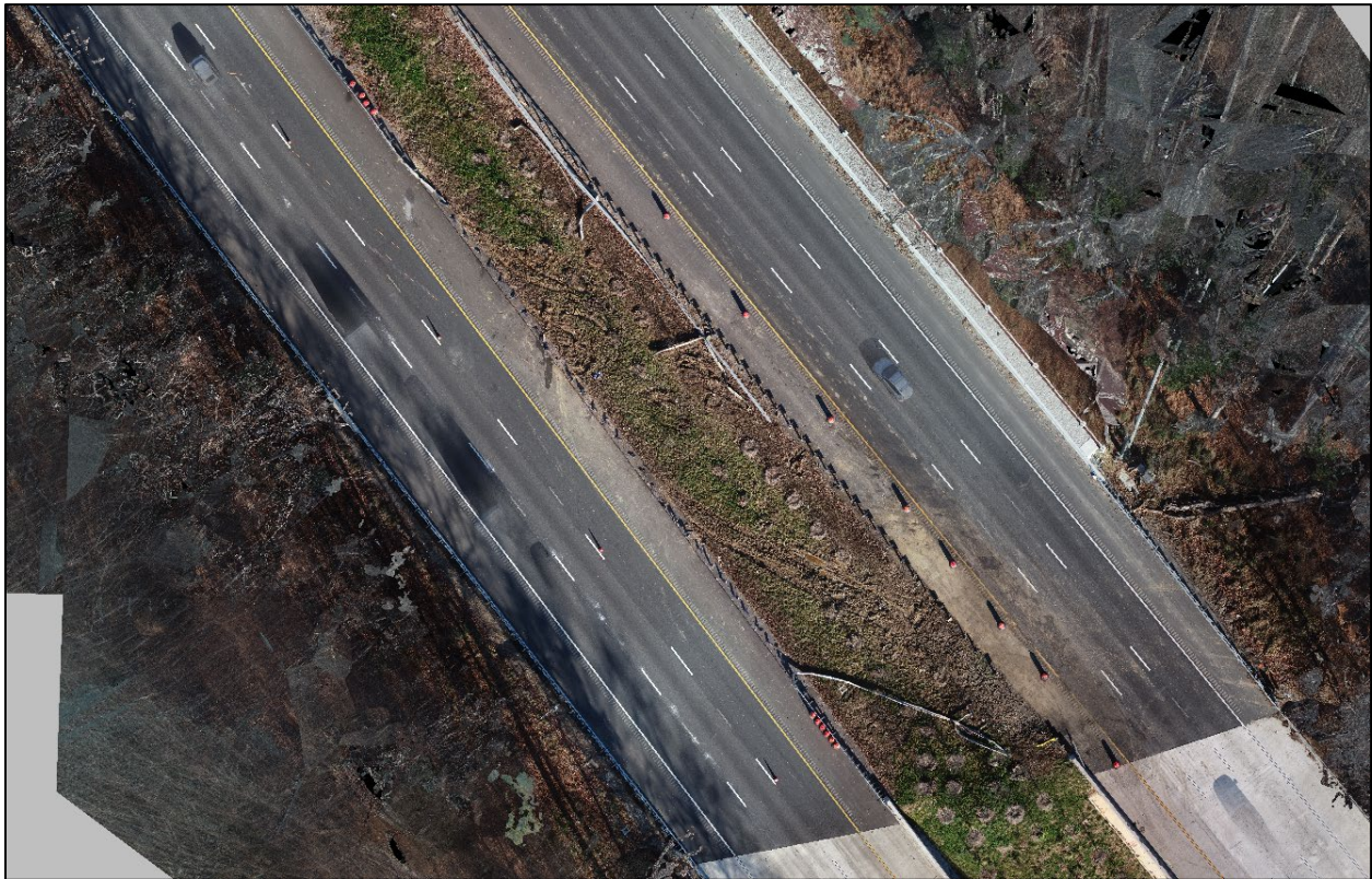
Figure 3: Screen capture depicting a portion of the photogrammetry project orthomosaic image capturing road surface and median evidence as well as the displaced eastbound shoulder guardrail.
