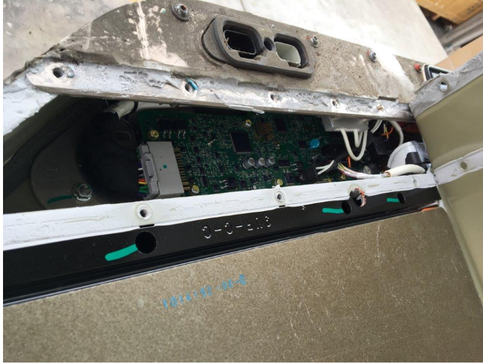
Burbank Inspection Photo 43: removing battery case cover at rear
