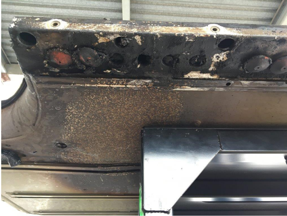
Burbank Inspection Photo 27: view showing left side front vents, after cover has been removed
