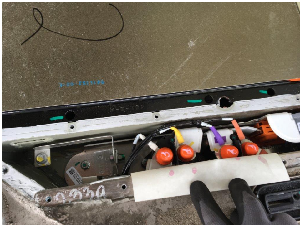
Burbank Inspection Photo 44: aft access panel with cover removed
