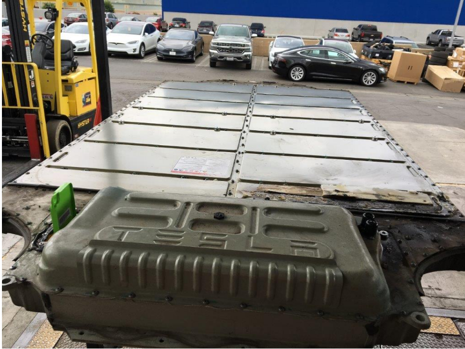
Burbank Inspection Photo 33: battery case top front view, plastic cover removed
