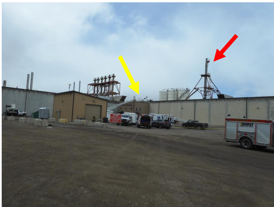
Photo 2: Photo of the smokestacks on the Gem State Processing building. The red arrow indicates the stack that was struck by the accident airplane, and the yellow arrow indicates where the wreckage was located. The airplane was traveling right to left in the photo. 55
