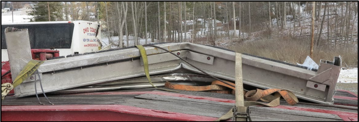
Photograph 12: Looking at the damage to the steel frame from above the cargo doors on the 2019 Hyundai semitrailer.
