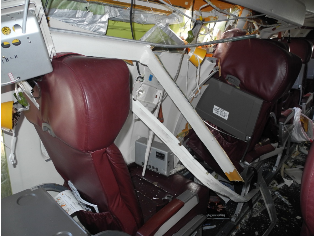
Photo 8. Interior damage above seat 5A.
