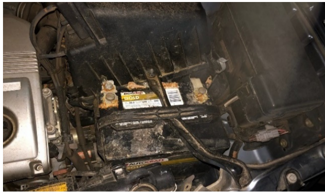
Heavily corroded battery with terminals still connected found in vehicle on Ro-Ro, taken in June 2020, provided by the Coast Guard.
