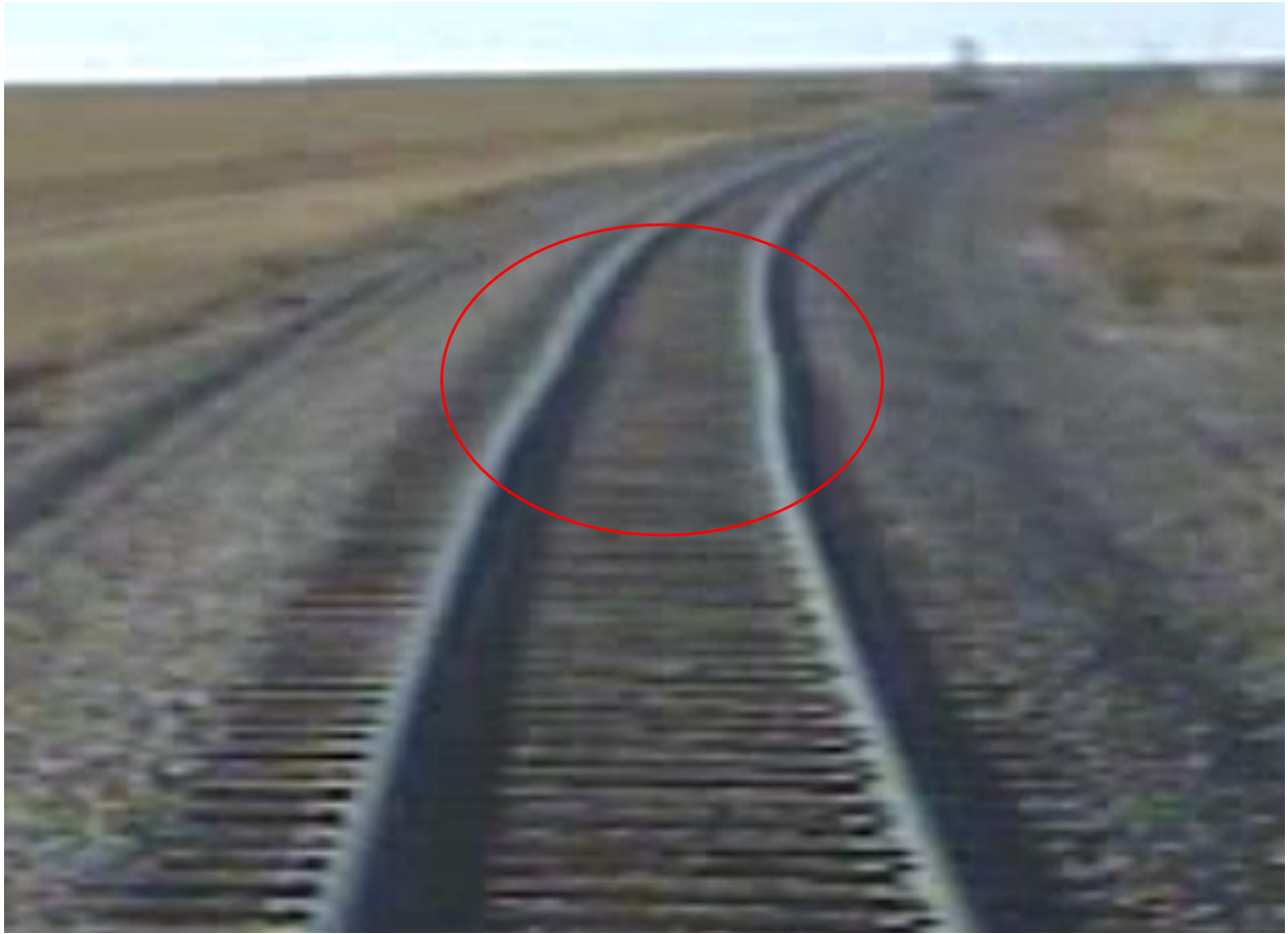
Figure 5- Head-end of Amtrak train No. 7 showing misaligned track
