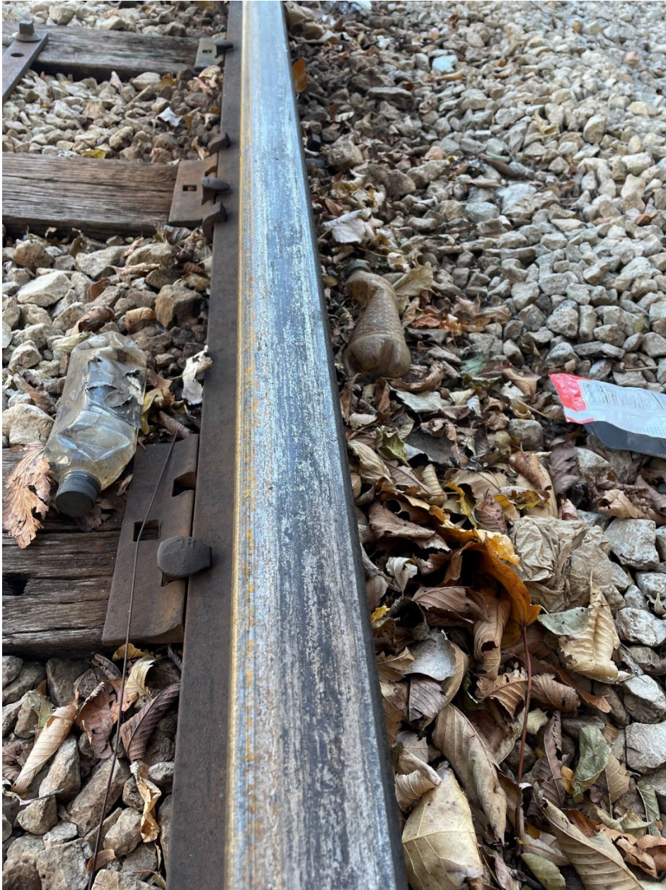
Figure 3: Photo of black substance found on top of the rail. (Source: NTSB)
