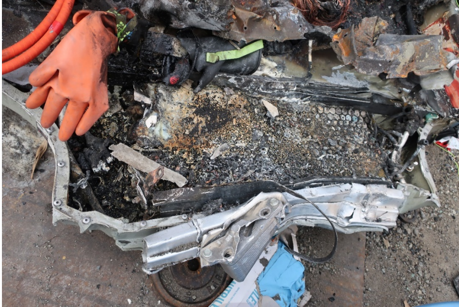
Figure 17. View of front of the 400 VDC 100 kWh battery, as found, looking down and aft. The black and red rubber gloves are on the 14 positive bus bar. The exposed cells are the tops of module 15 and the buckle through the middle of module 15 is visible.
