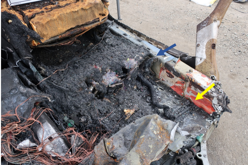
Figure 7. Fire damaged wiring in lower left. The driver seat is at top left of driver footwell. The lower yellow arrow shows the remaining forward edge of the vapor barrier. The step-like appearance at the upper blue arrow is the edge of the egg crate foam beneath the carpet.
